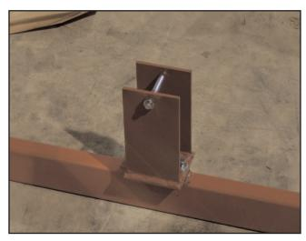
Attach Support Beam Mount to Support Beam with supplied bolts. Tighten securely.
