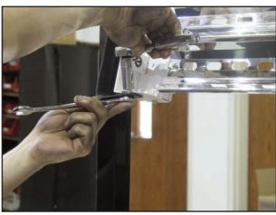
Fully tighten all nuts on brackets (included and already pre-assembled) on Light Housings (C).
