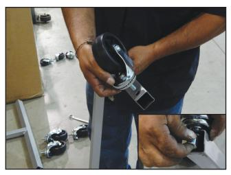
Insert wheel into the support base. Place the washer and nut onto the wheel bolt. Tighten the nut. Repeat for other 3 wheels.
