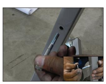
Insert the bolt into the bottom hole on one of the support bases.
